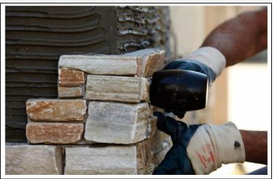
12.2 Starting with a long-cornered panel, the bottom row of panels is placed into position supported by either a plinth or a profile made from aluminium or stainless or galvanized steel. A rubber mallet may be used to help consolidate the mortar adhesive and align the panels. The end panel is trimmed to fit using a suitable tool such as an abrasive disc. The process is repeated for each row, ensuring that joints are staggered (eg by alternate use of long- and short-cornered panels).
